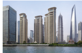
Tomson Riviera Apartment Towers Shanghai, China
